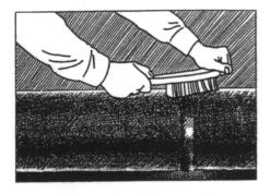
Clean any loose scale or rust from the selected attachment area. Do not clean to bright metal. Also, never use a powered grinding tool as this can damage the weld.
