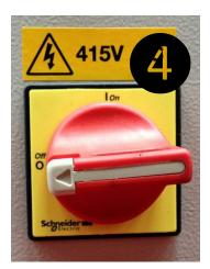
Also, on the door of the control panel is an Electrical Isolation Switch **4**. The switch must be turned to the off position, cutting power to the panel in order to open the door. The handle can also accept a padlock or similar, in order to lock out the panel and prevent it from being powered up.
