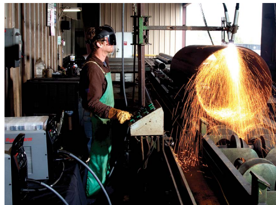
Pipe cutting and beveling
