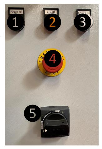
If there is a fault, or the emergency stop is active, then the alarm lamp **2** will illuminate. This must be cleared before operating the positioners.
