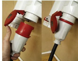
Plug the welding earth cables into the controller. Note that the cable end weld plug has a peg which mates with the key slot in the panel mounted socket.
