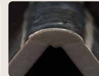
A stable arc ensures a smooth weld and strong base material attachment, thus ensuring good mechanical properties for the joint.
