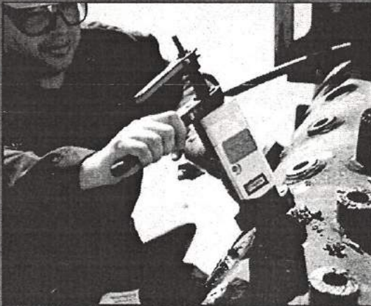
Solution Profile: The rugged BOILERMASTER™ being used to rapidly face header stubs which had been torch cut.
