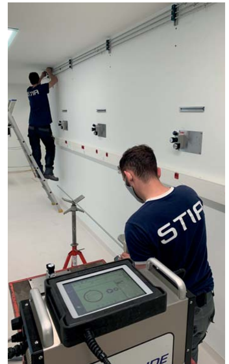
Figure 2. On-site installation for medical gas lines in a hospital.
