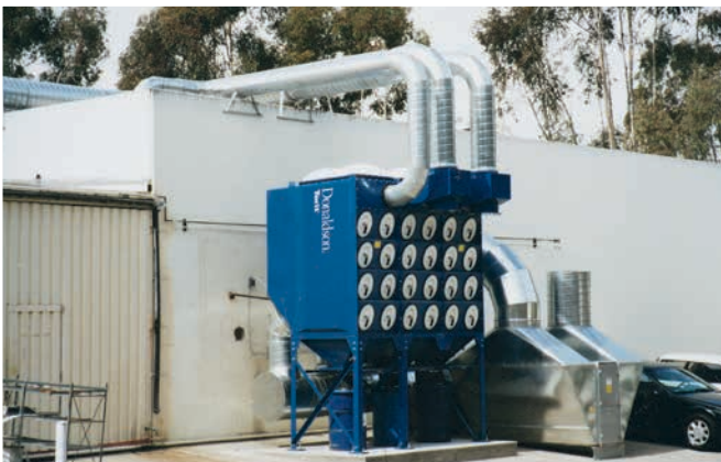
DFO 4-48 on Metal Grinding
