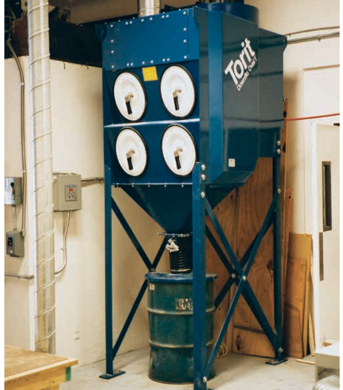
DFO 2-4 on Fiberglass Routing & Cutting
