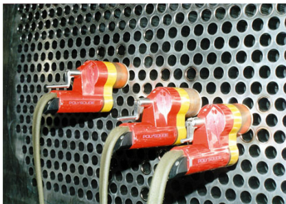
TS 25 in the production of heat exchangers
